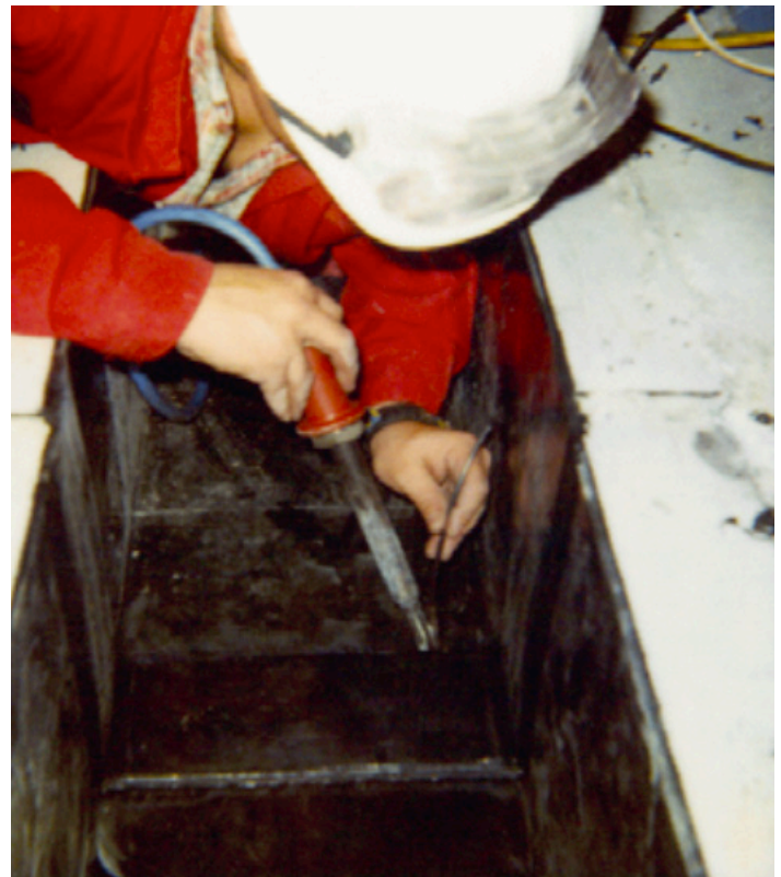
Joints between prefabricated trench liner sections are welded for leak-tight seal
